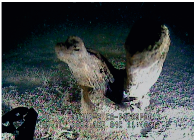
Figure 1 Hole with Protruding Material from Initial Inspection
