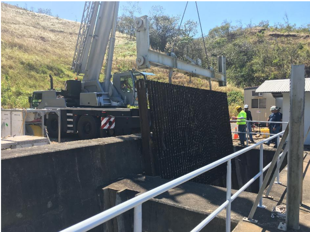
Figure 10: Retirada das grades
