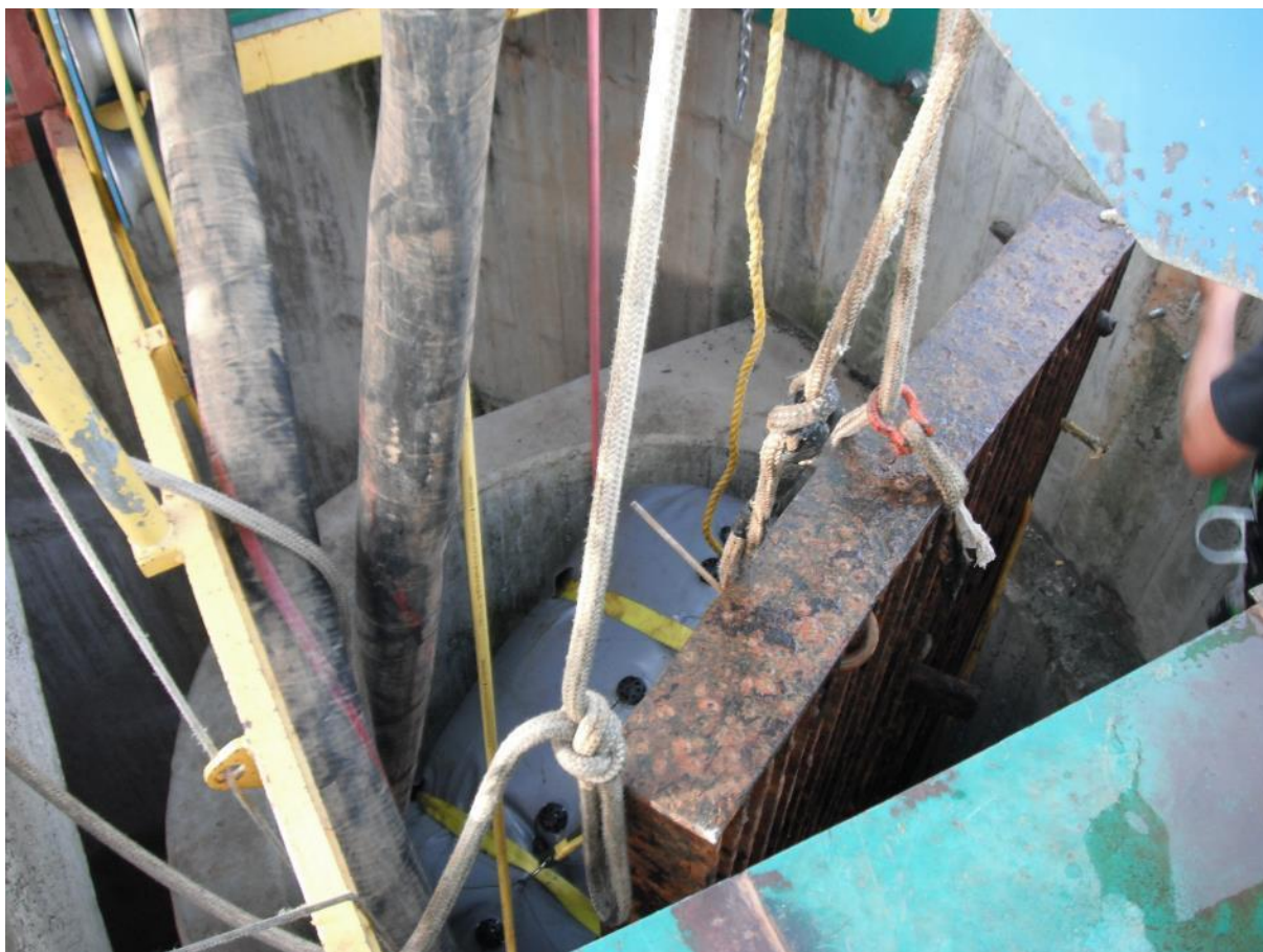
Figure 6: Retirada das grades
